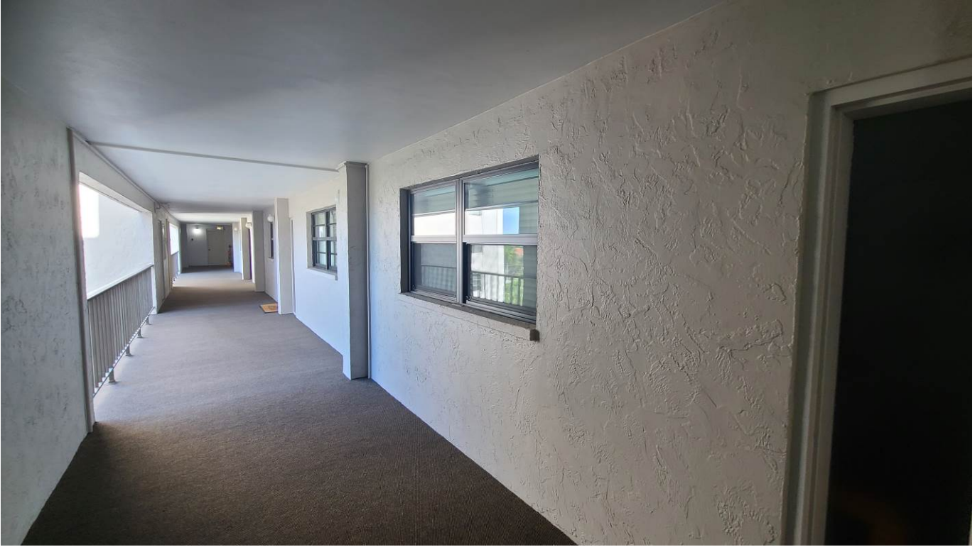
Photograph 15: Building Walkways – Current Condition.
