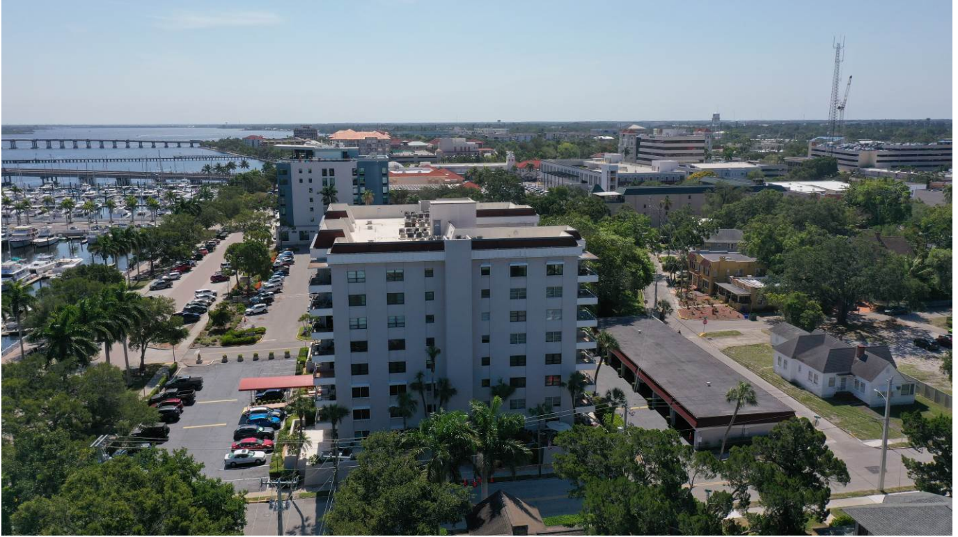
Photograph 3: View of the East Elevation of the Building.
