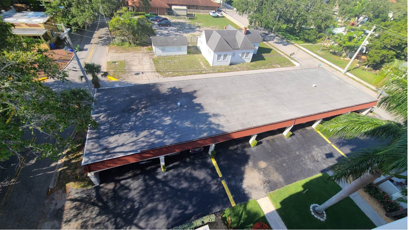
Photograph 22: Building Common Areas – Carport
