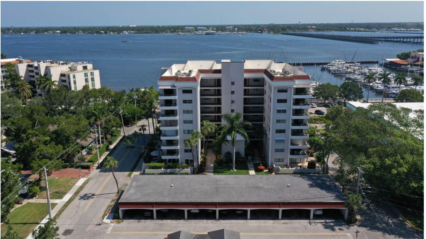
Photograph 2: View of the Rear (Back) Elevation (South).
