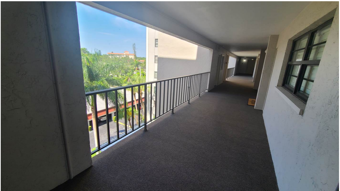
Photograph 14: Building Walkways – Current Condition.
