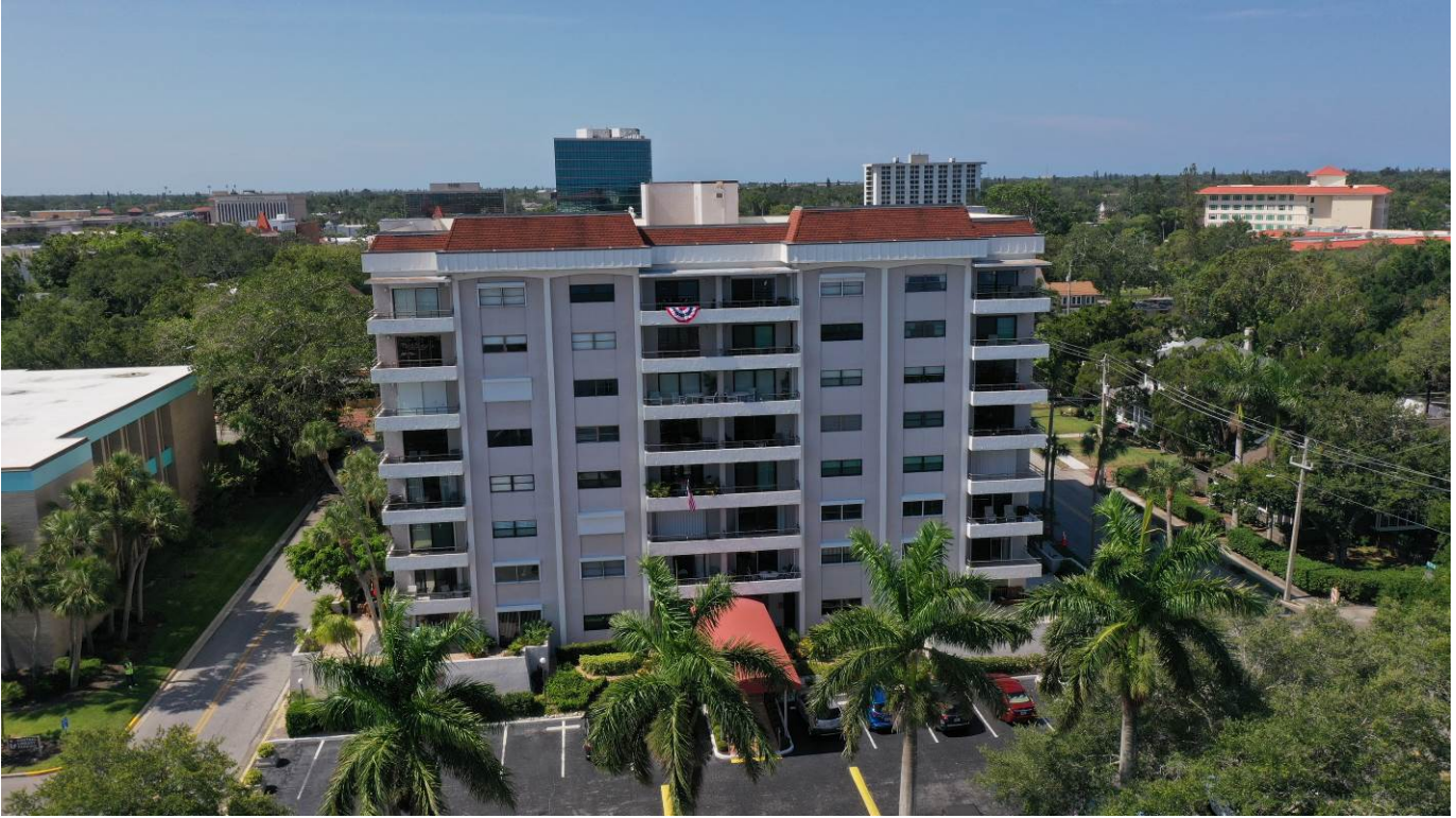
Photograph 1: View of the Front Elevation (North).
