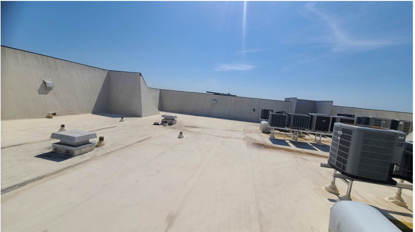
Photograph 8: The Roof, Current Condition.
