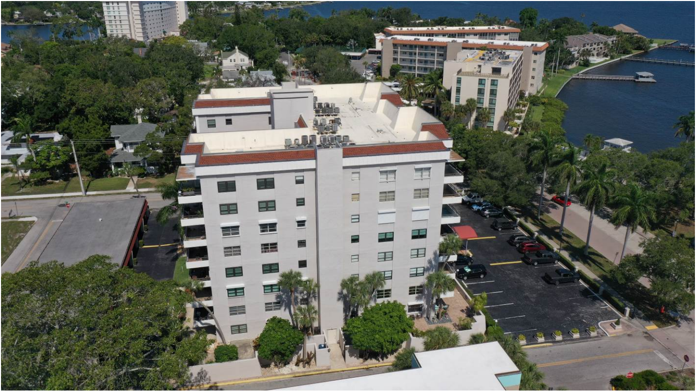
Photograph 4: View of the West Elevation of the Building.
